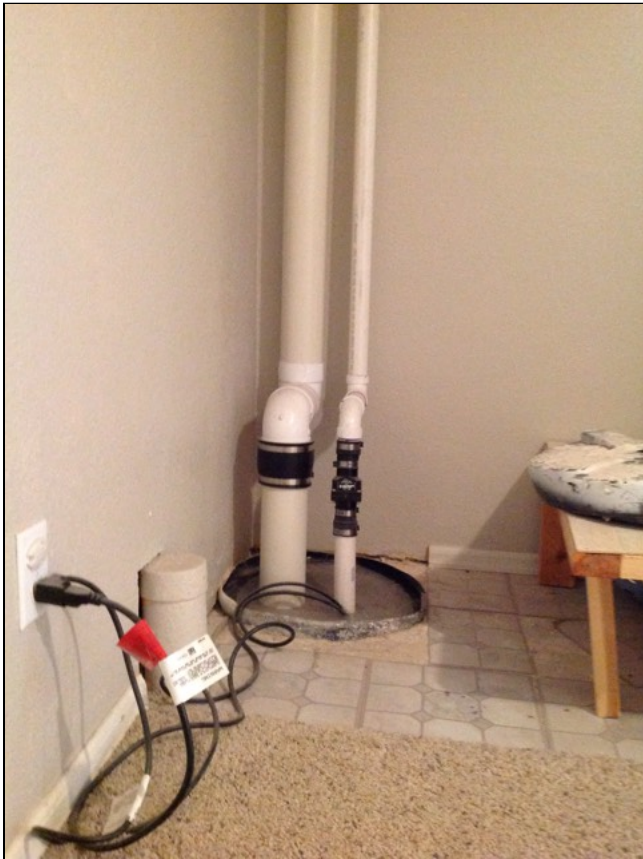
5.6 Item 1(Picture) Basement level near left side facing front of house
