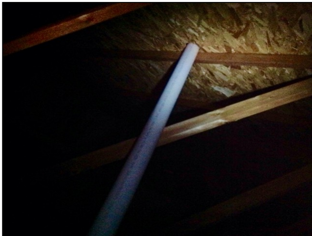
1.2 Item 5(Picture) Plumbing vent pipe.
