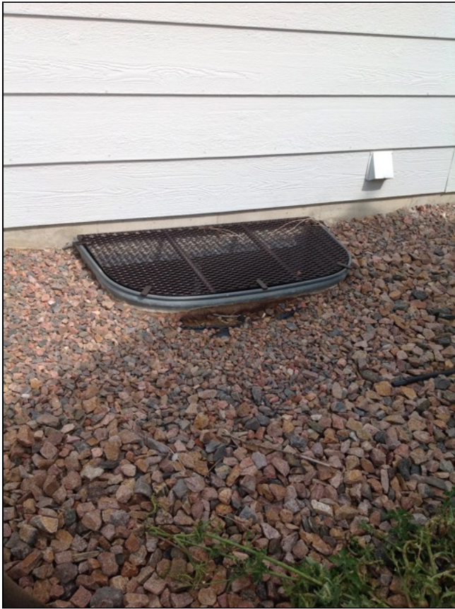
2.2 Item 3(Picture) Window well at left side facing front of house.
