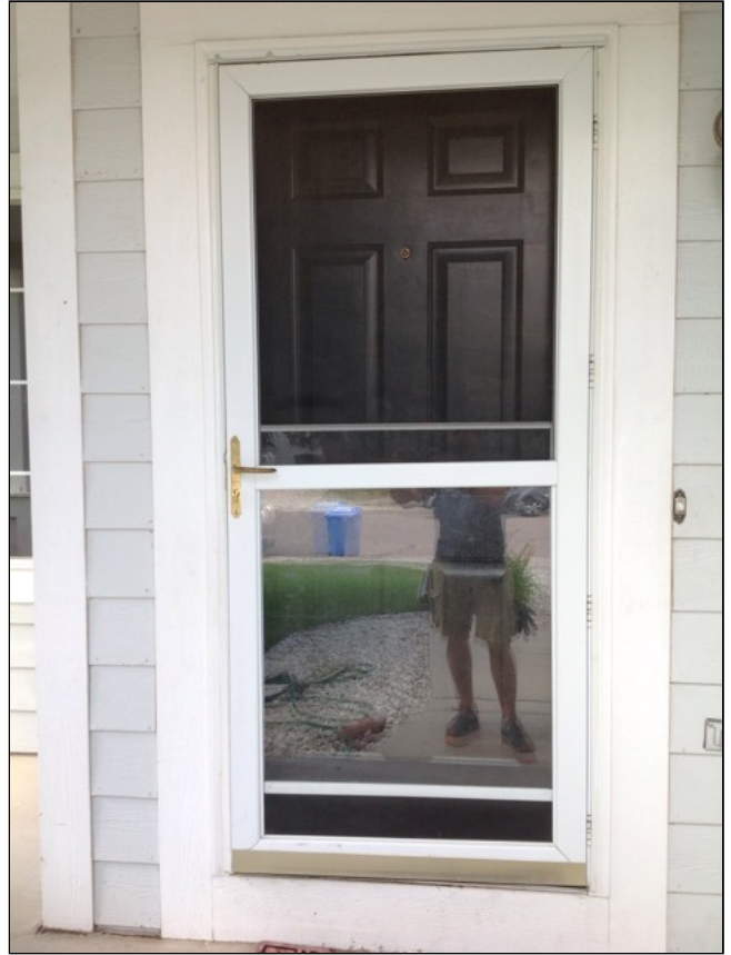
2.1 Item 2(Picture) Front entryway storm door.
