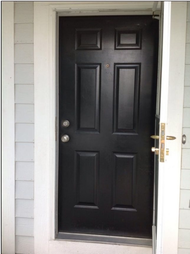
2.1 Item 1(Picture) Front entry doorway.
