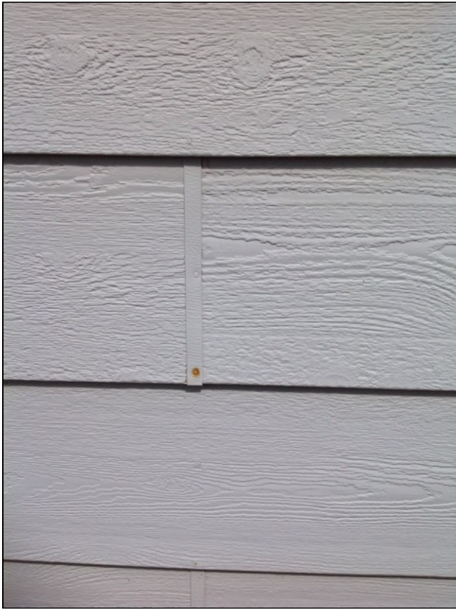
2.0 Item 1(Picture) Rusty nail heads present at left side (facing front). Repair as needed.
