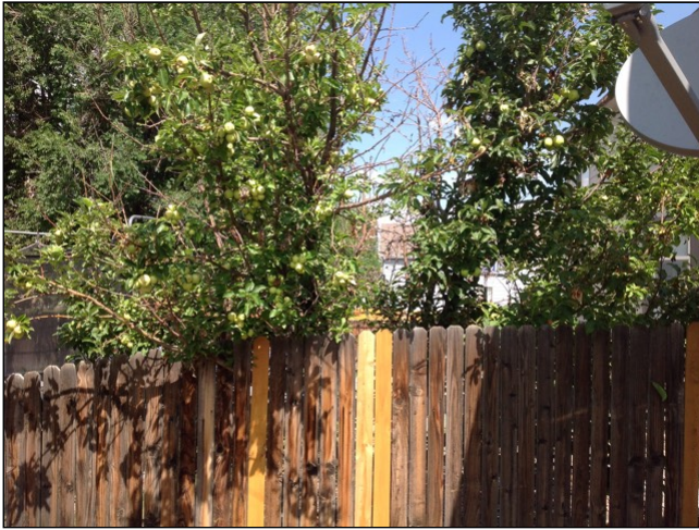
The tree limbs that are hanging near the neighboring house should be trimmed. Potential rubbing of siding and roof could occur.
