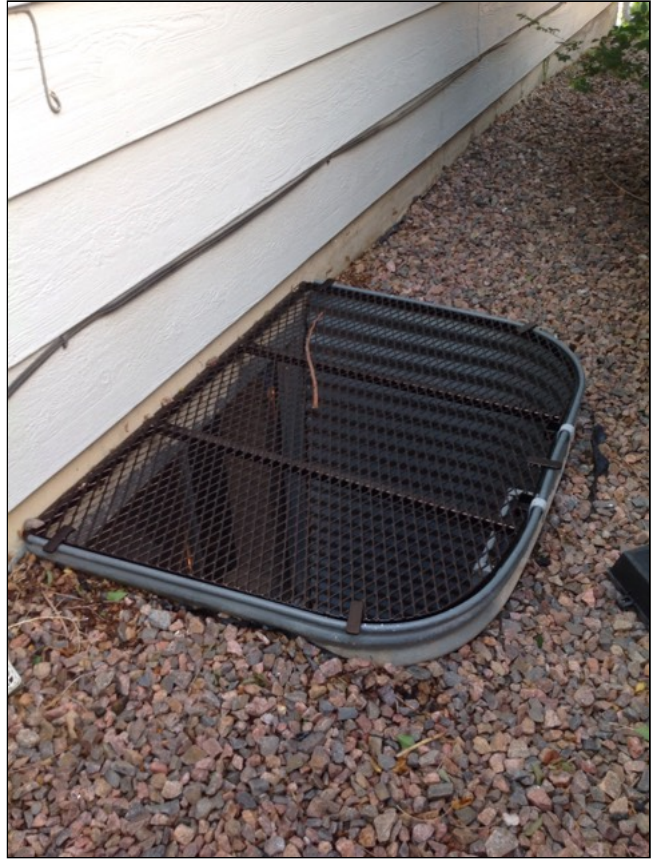
2.2 Item 2(Picture) Window well at right side from front of house
