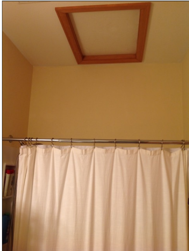
1.2 Item 4(Picture) Attic space access from main level bathroom.
