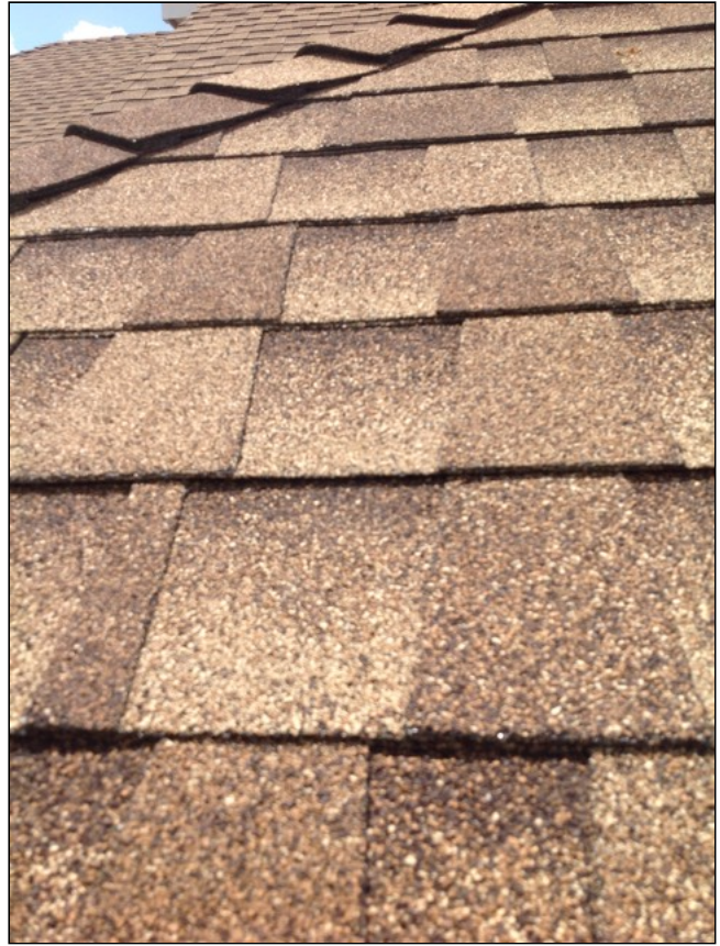
Single layer 3-tab shingles. No fasteners sicken or protruding.
