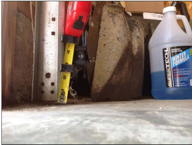
9.5 Item 2(Picture) Sensors positioned correctly and operable when tested.
