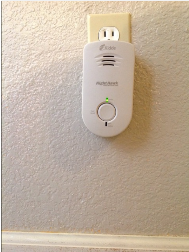
6.9 Item 1(Picture) Located in hallway 1st level.
