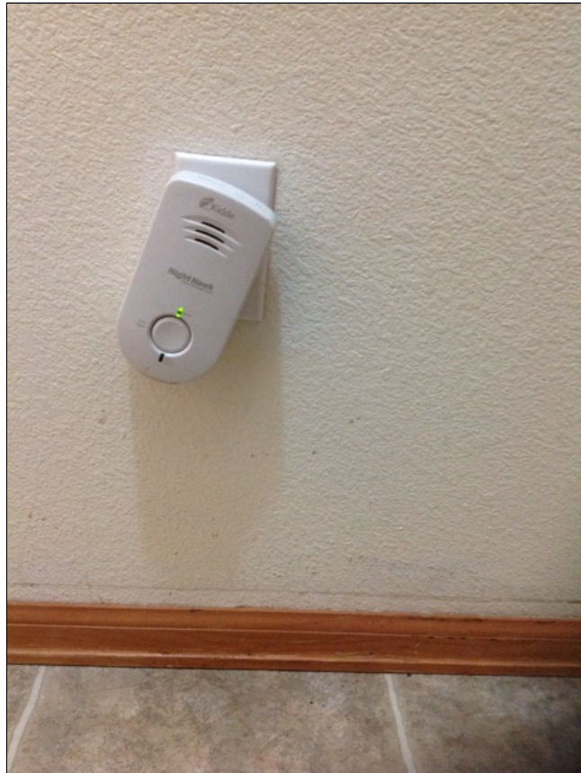
6.9 Item 2(Picture) Located lower level basement.
