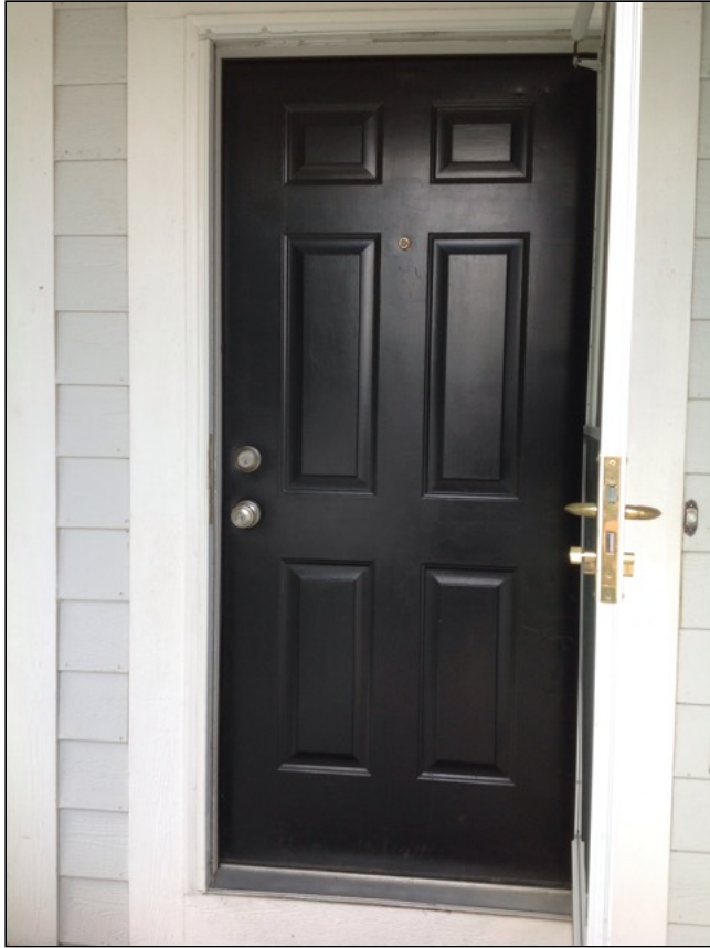
2.1 Item 1(Picture) Front entry doorway.
