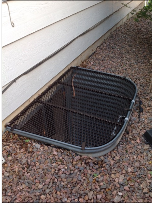
2.2 Item 2(Picture) Window well at right side from front of house
